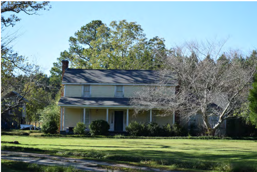
Cutler House (BF1595), view to the southwest
