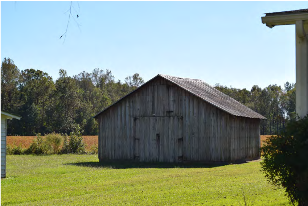
Board-and-batten circa 1920 barn, view to the southeast
