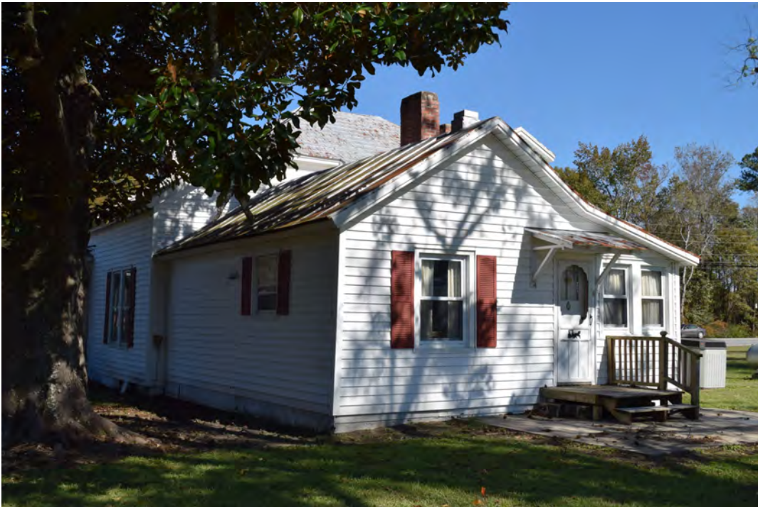
Southwest corner of rear ell, view to the northeast
