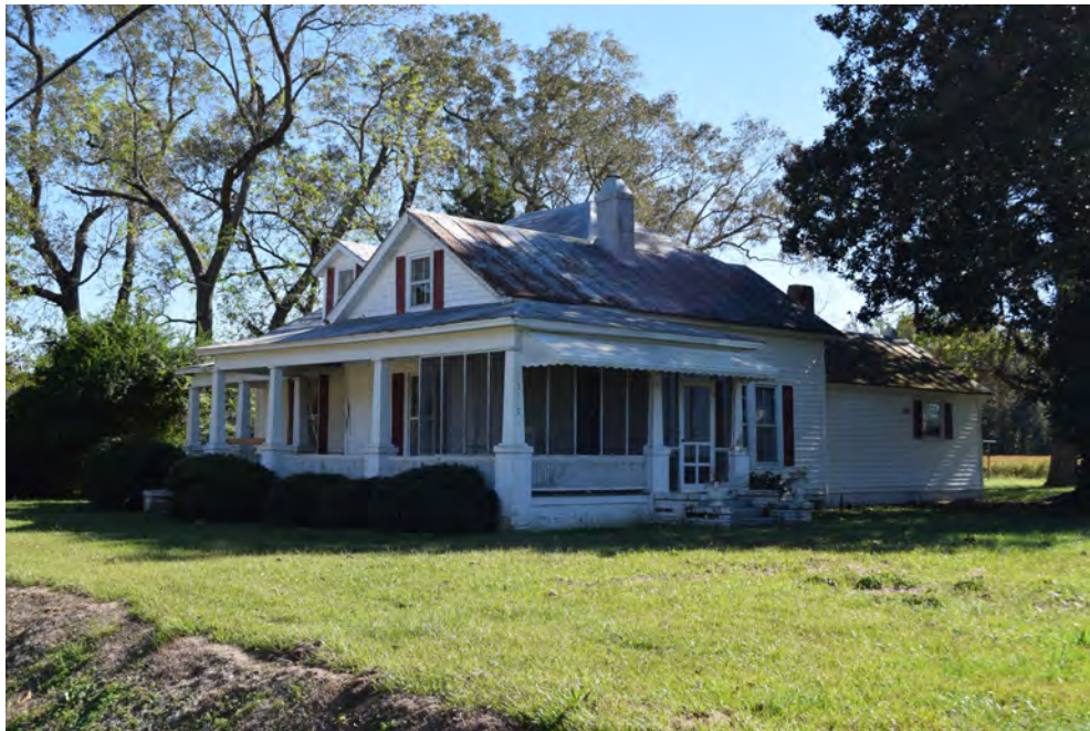
Northwest (front) corner of the Mixon House, view to the south
