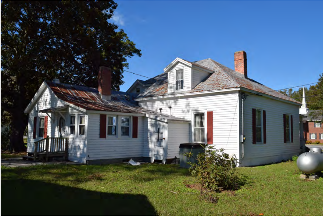
Southeast corner of the Mixon House, view to the north
