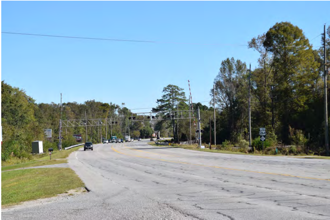
US 264 at the beginning of project area at Alfen Lane, view to the southeast
