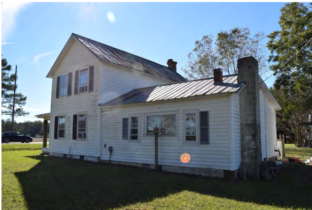
Northeast (rear) corner, view to the southwest
