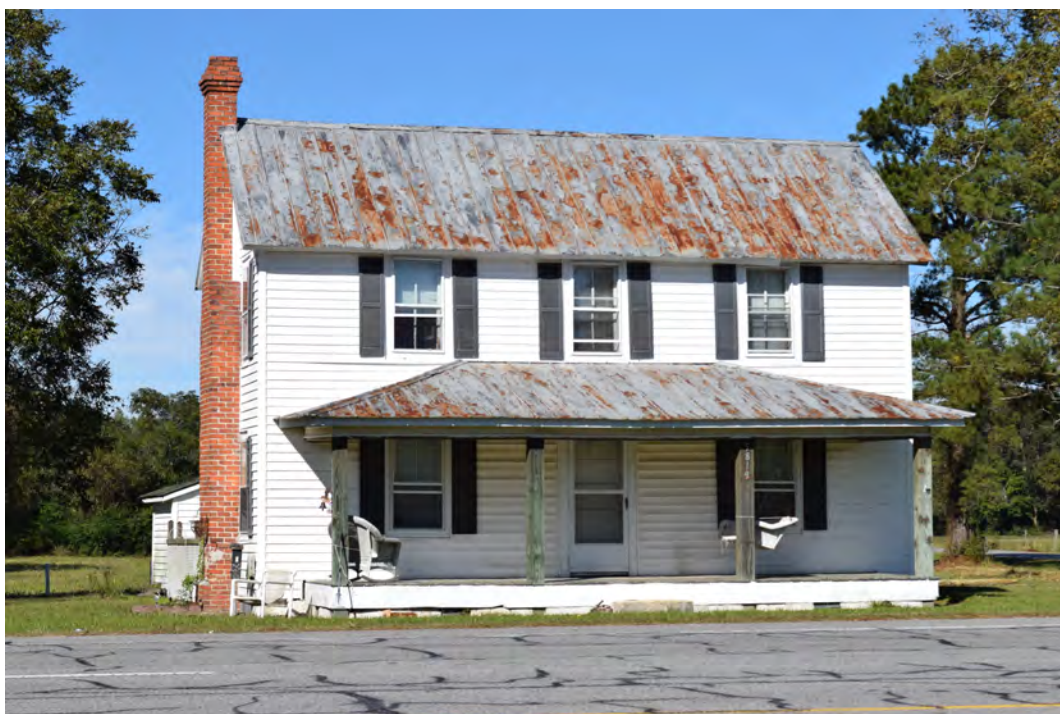
Façade, view to the north
