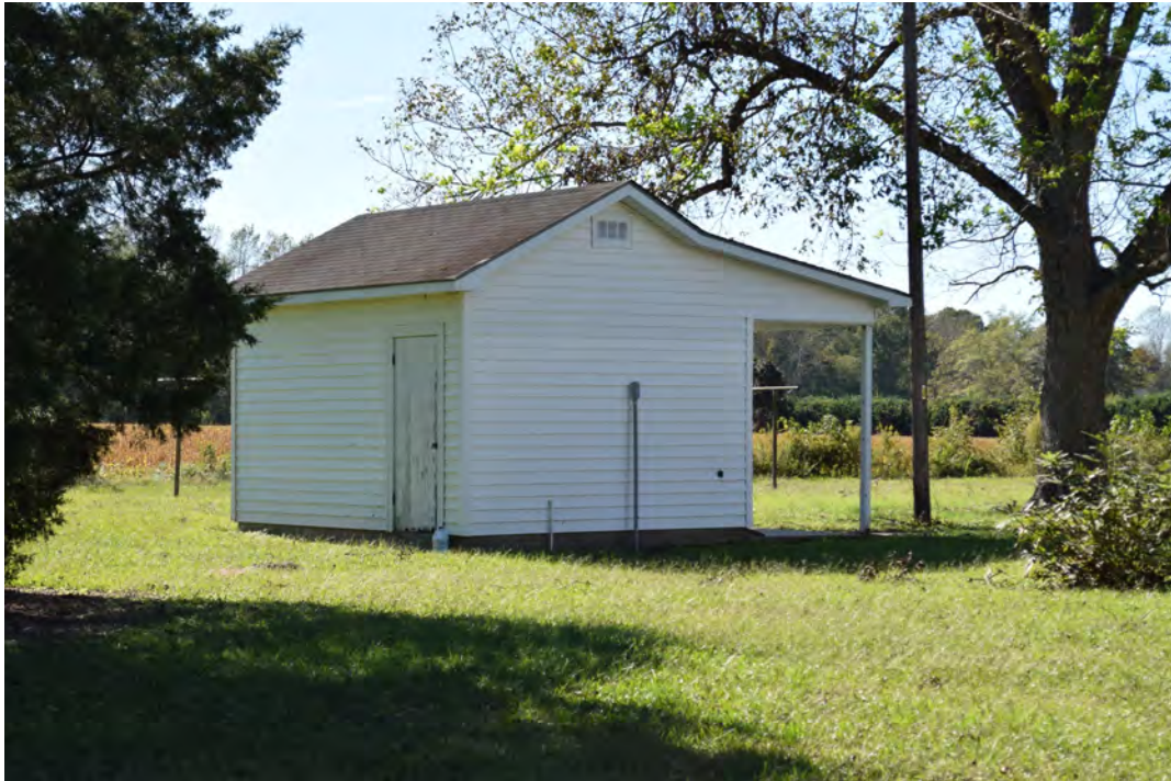
Vinyl-sided workshop from circa 1970, view to the southwest
