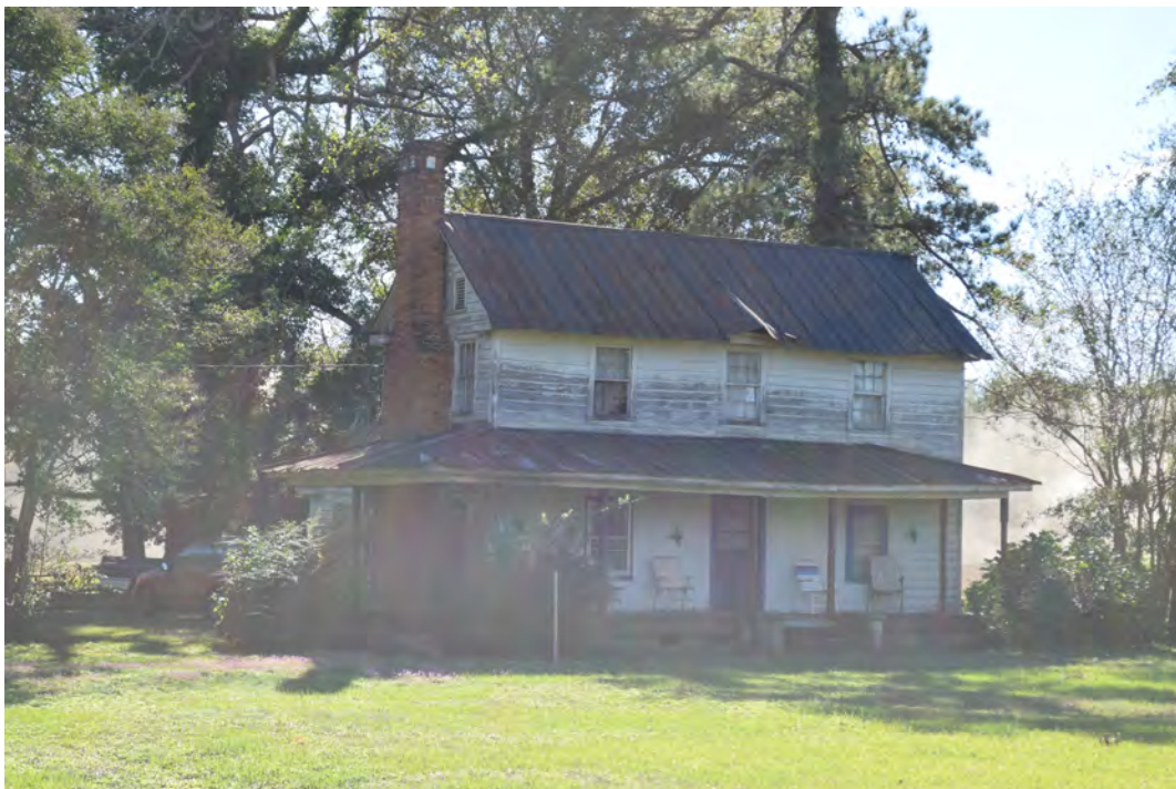
House (BF1474) at 32 Camp Leach Road, view to the southwest
